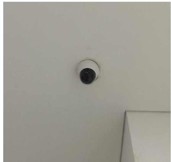
Figure 20 Dome Camera
