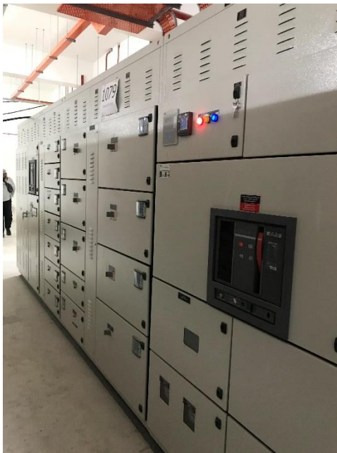
Figure 27 Tenant Main Switchboard
