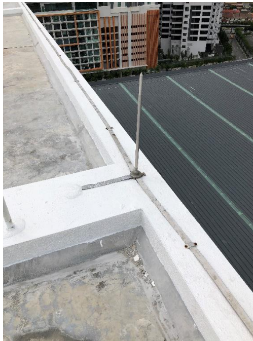
Figure 30 Air terminal on the rooftop
