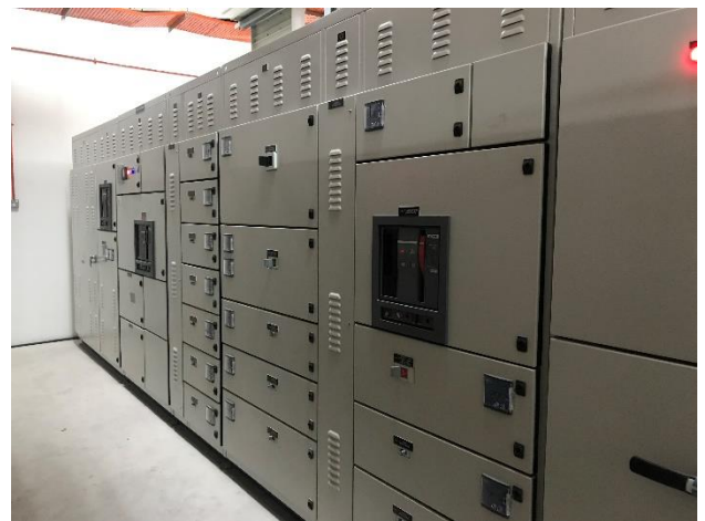
Figure 28 Landlord Main Switchboard
