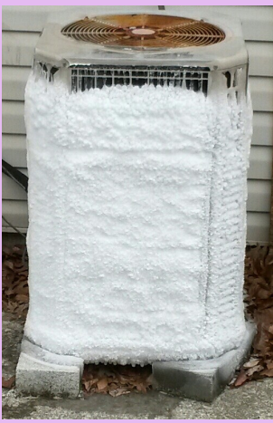
Frost formed on heat pump
