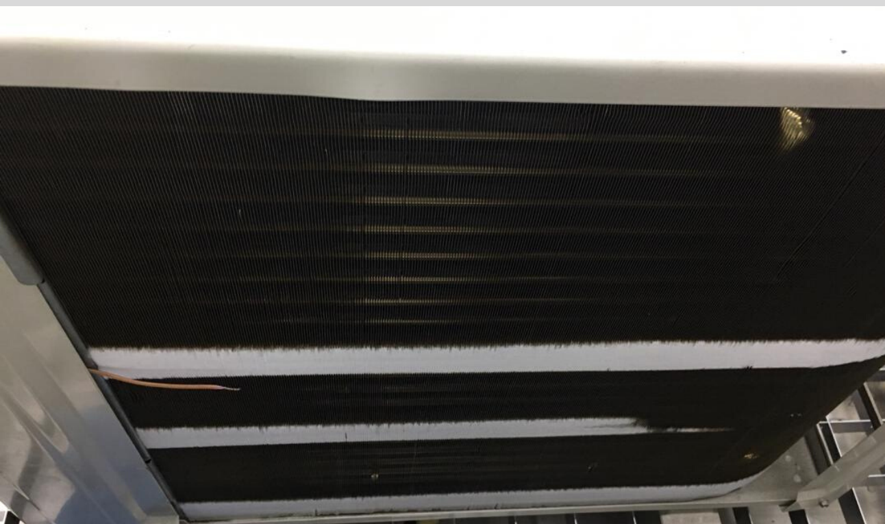
Frost formed on heat pump
