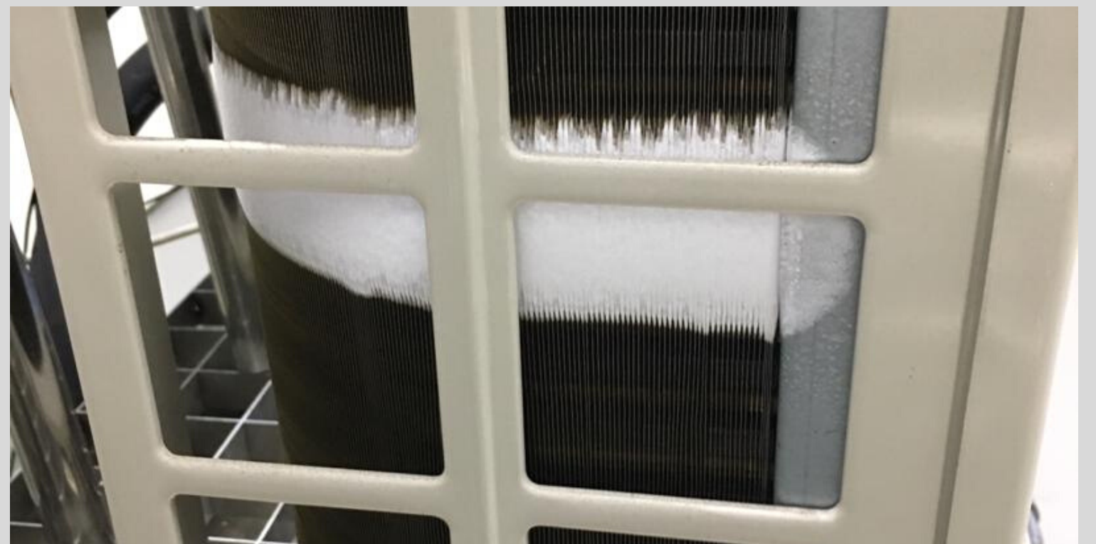
Frost formed on heat pump
